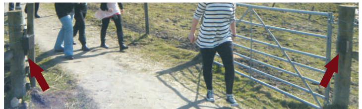
Protective Housing on gate posts
